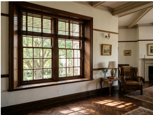
Original rooms. Wooden slats inside a deep reveal read as part of the joinery.
